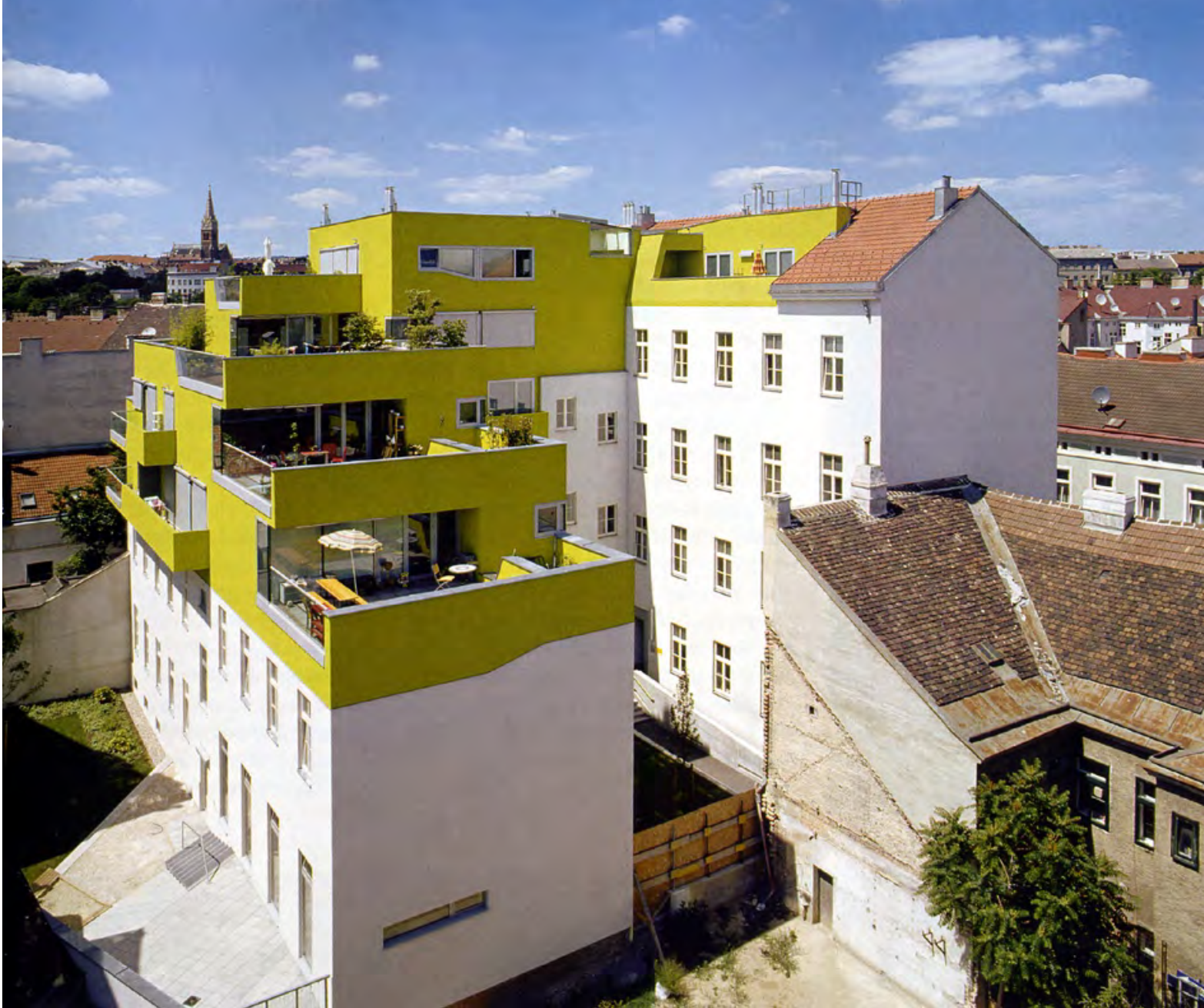
Bloc renewal | Roofextension | SIGGS Bauplanung | Sperrgasse | 2004 |
