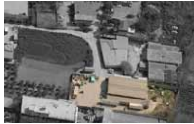
Pefkon st. General storage
