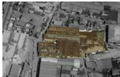
43 Knossou st. Metalworks
