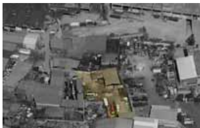
43 Knossou st. Metalworks
