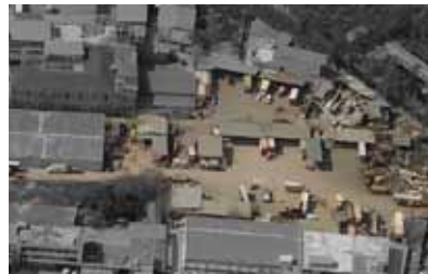
176 Orfeos st. Hauling station
