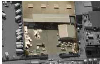
182 Leoforos Eirinis Av. Construction material storing
